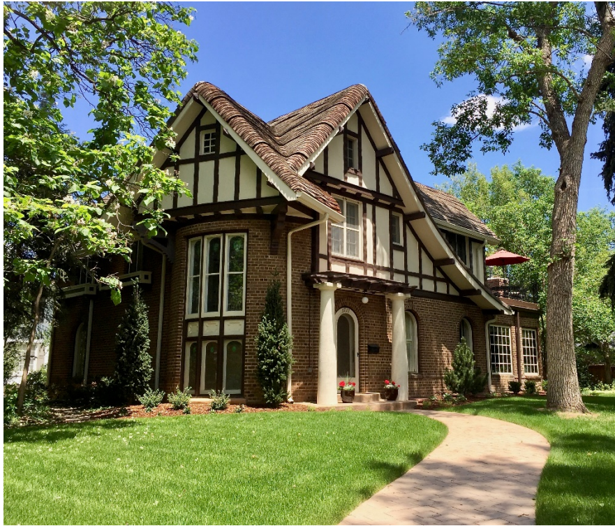
Figure 1 1717 E Arizona Ave, 2019
