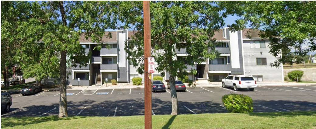
South of subject site, facing east from South Irving Street
