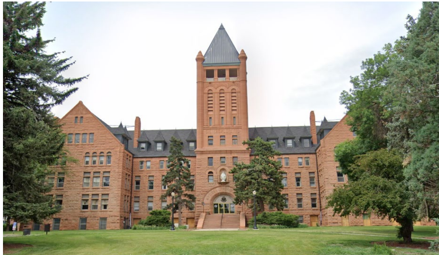
Subject site, facing west from former Loretto Heights Campus (Administration Building)
