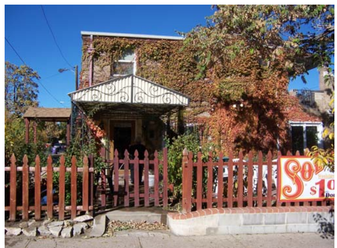
The adjacent property on the west.
