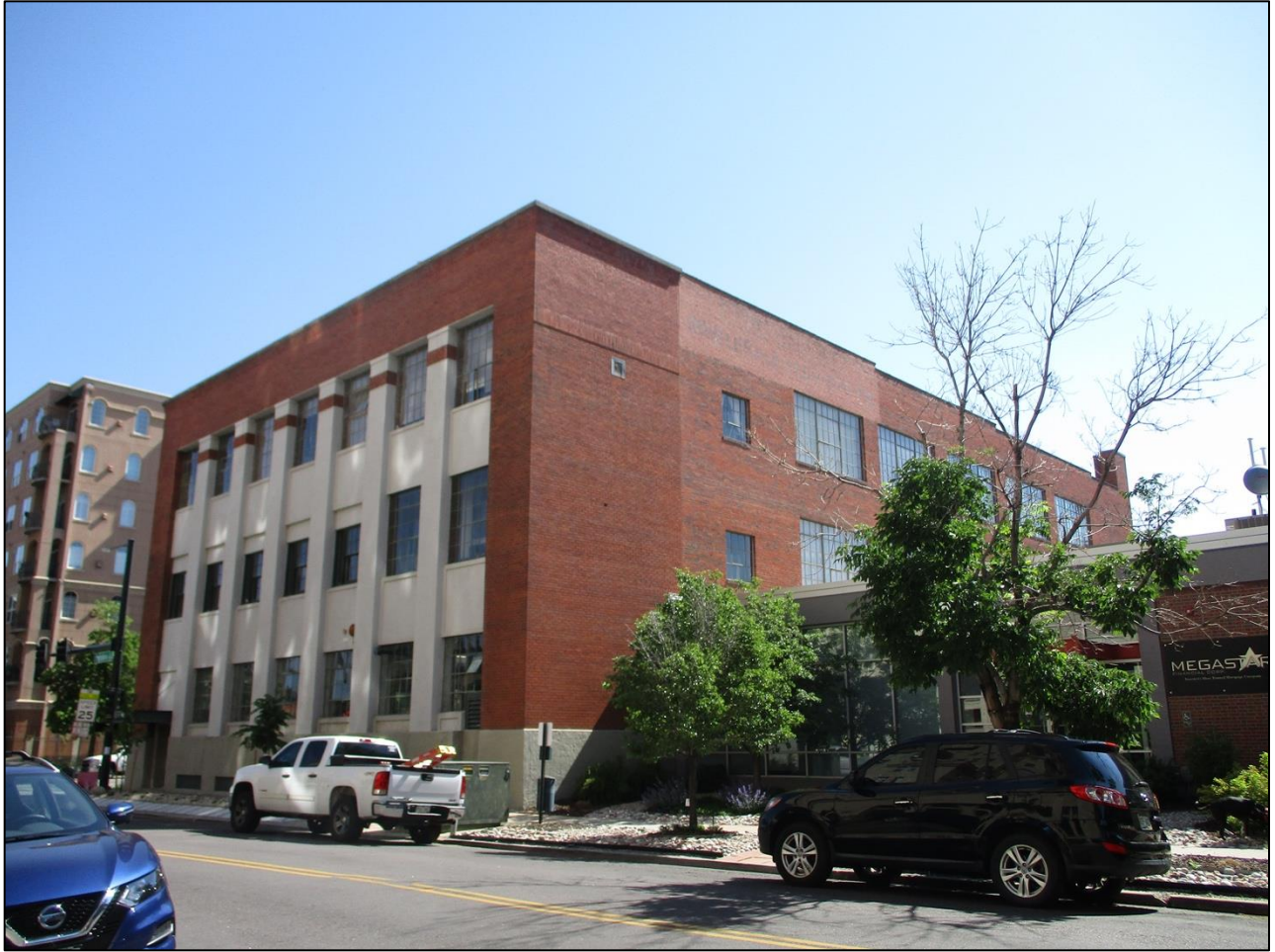
Looking northeast at west façade and south side
