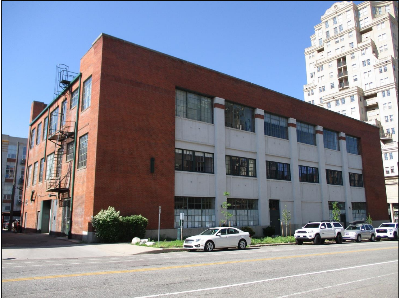
Looking southwest at north façade and east side
