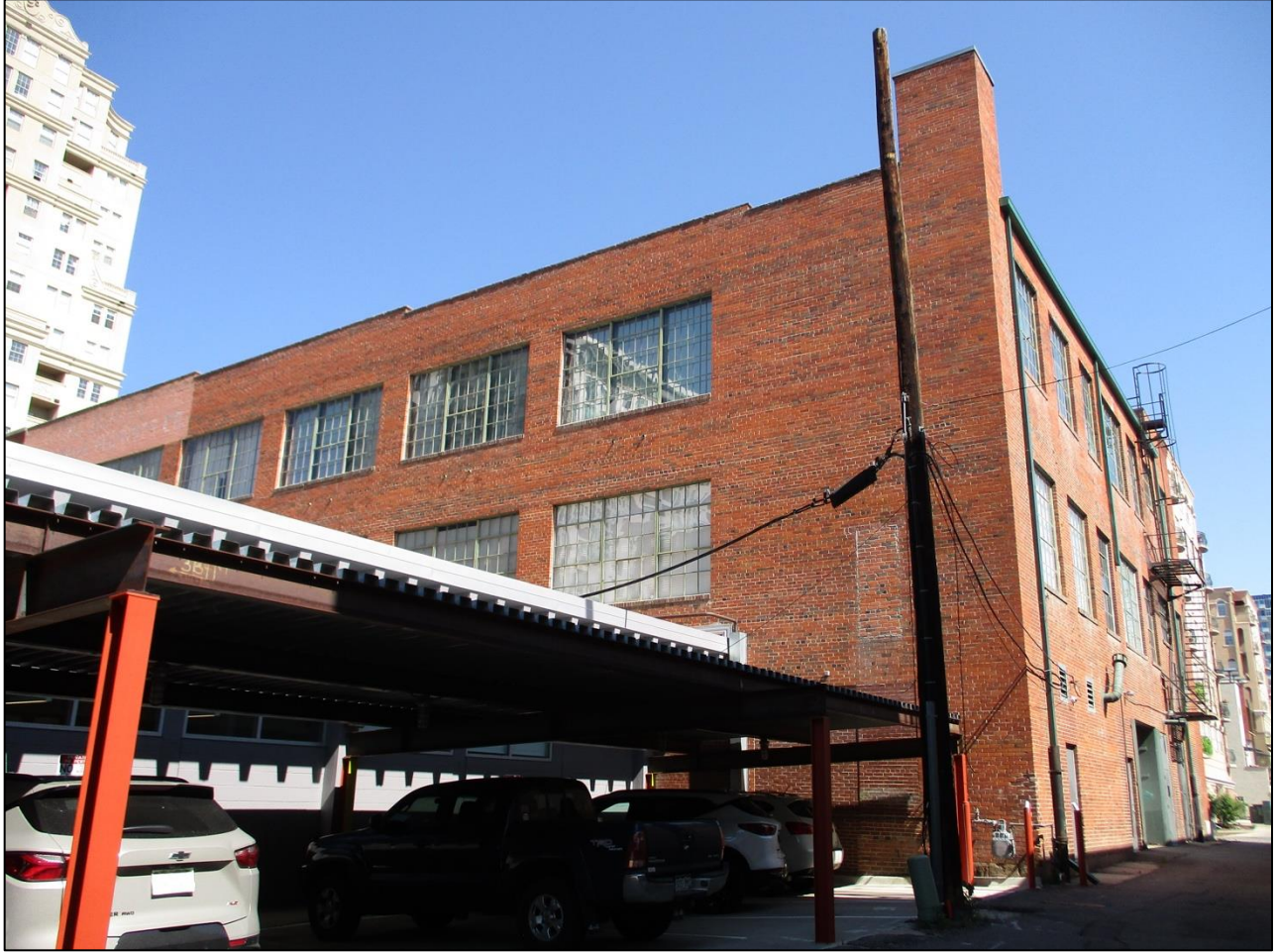
Looking north at south side
