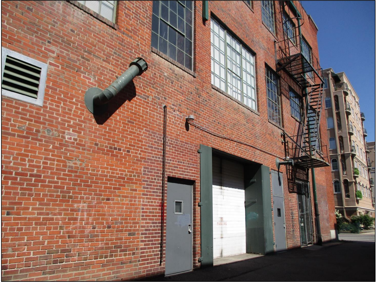
Looking northwest at exhaust pipes on east side
