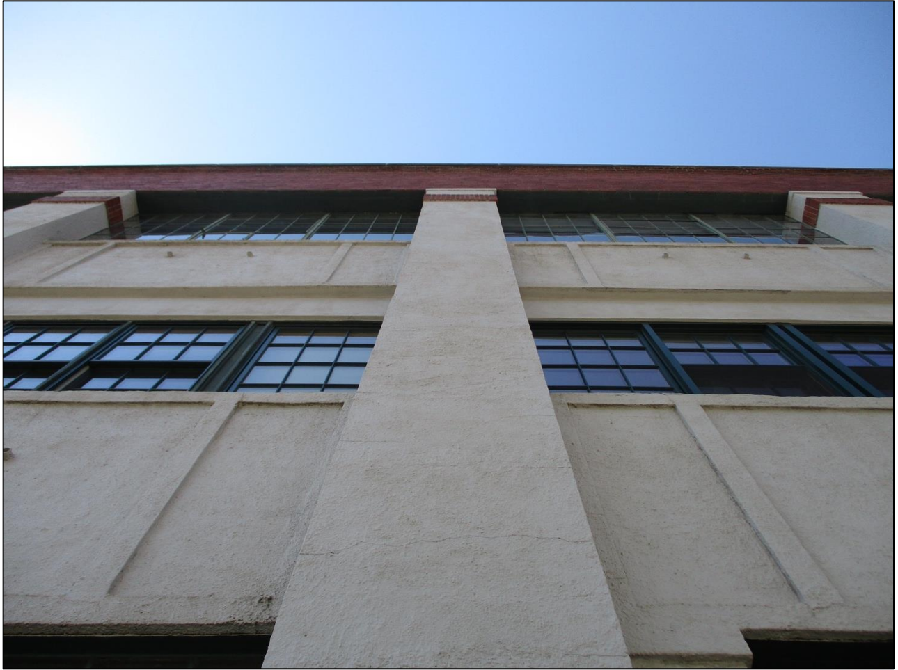
Looking up at north façade exterior
