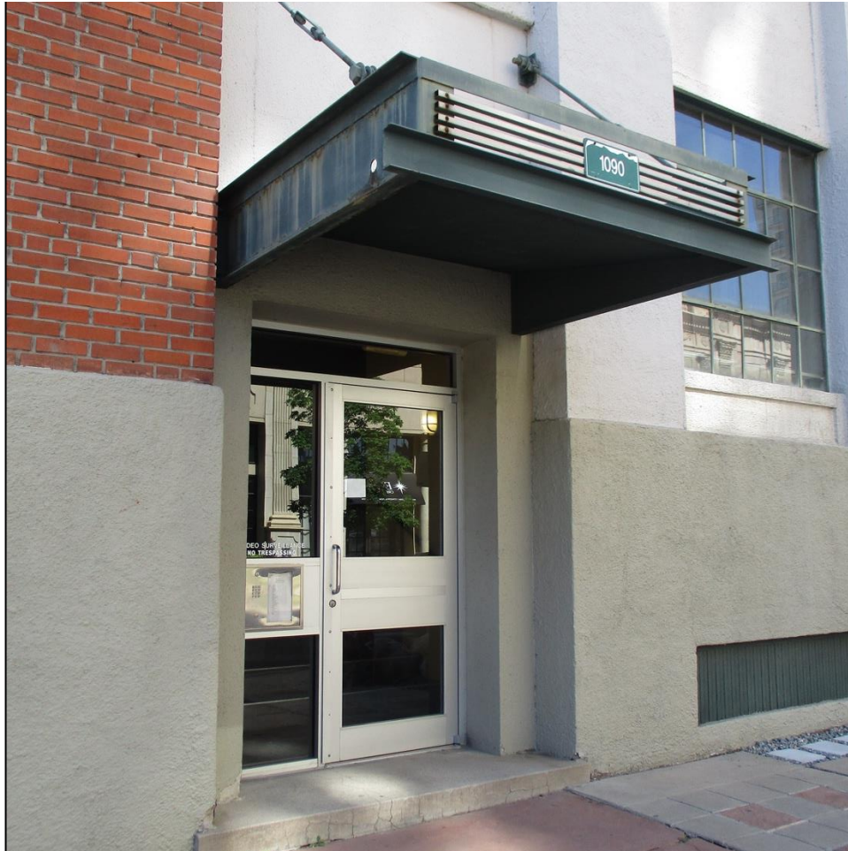
Looking southeast at main entrance on west façade
