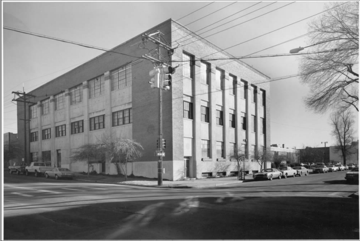
A vacant Cadillac Service Building in 1981; note alterations to some of the openings (Source: DPL Digital Collections, Z-10662)
