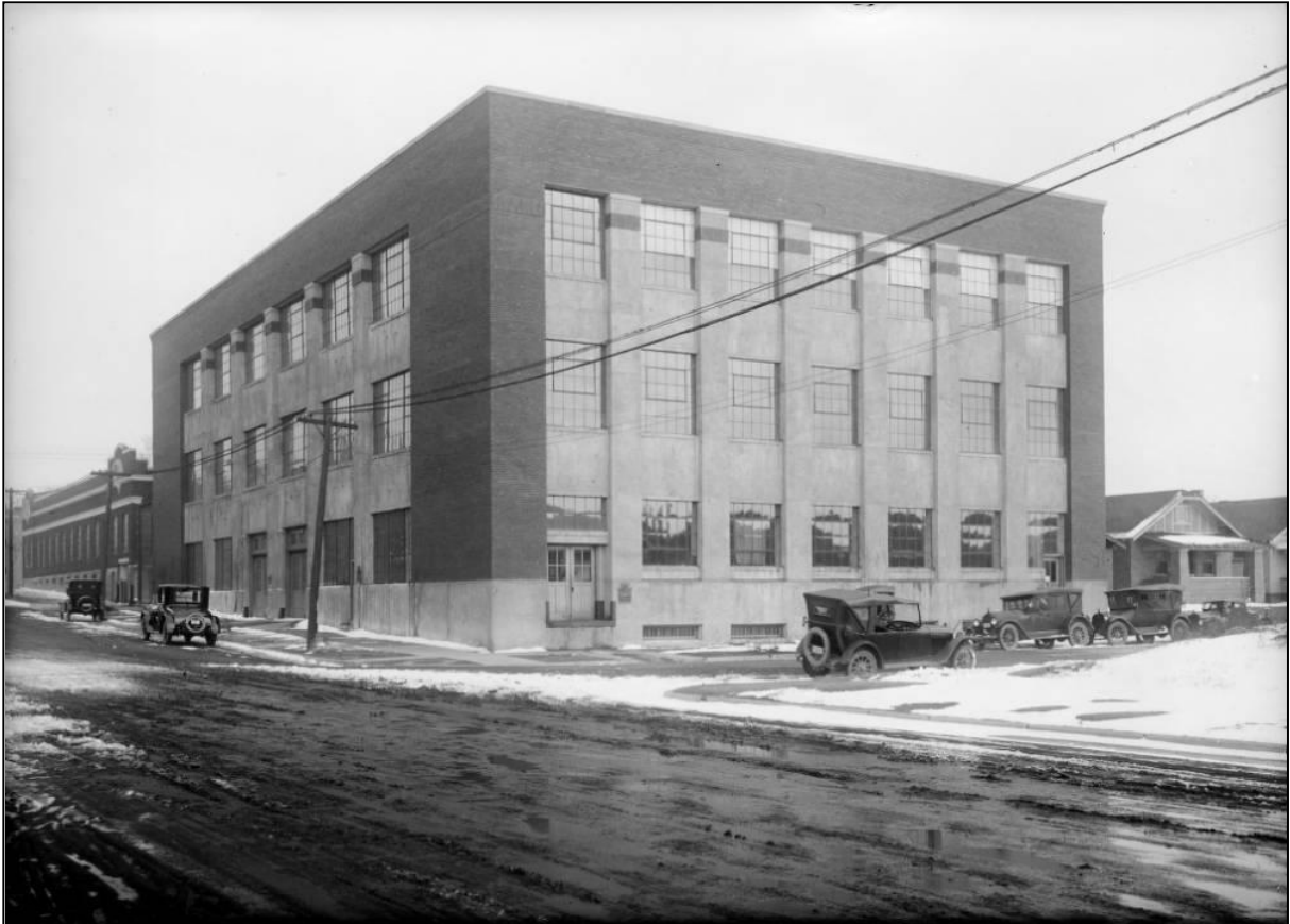
Cadillac Service Building between 1920-1930 (Source: DPL Digital Collections, X-23849)
