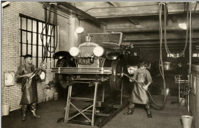
Cadillacs serviced in the building would have been cleaned on wash racks similar to this one (Source: Detroit Public Library's National Automotive History Collection, na042624)
