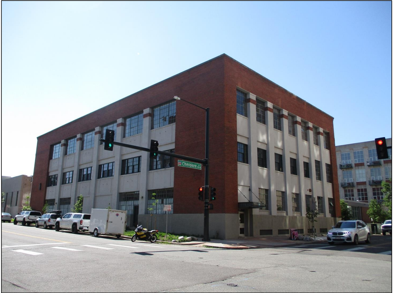
Looking southeast at west and north façades
