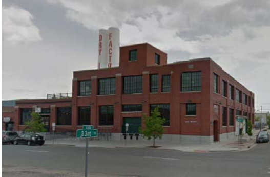
Office to the northwest of the site along Walnut St
