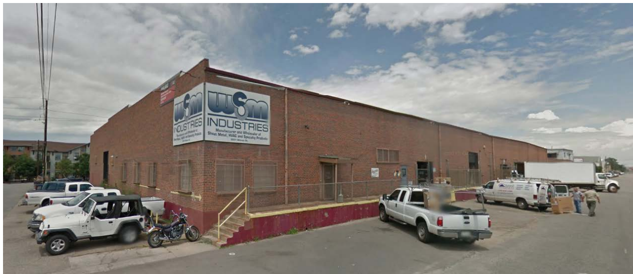
Subject site looking northeast along Walnut St.
