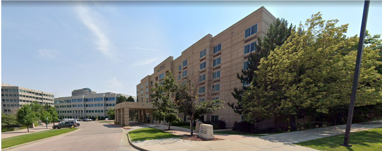
South – from East Bellevue Avenue (Source: Google Maps)
