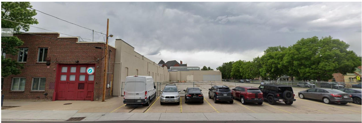
View of the subject property and existing building looking north from E. 35th Avenue.
