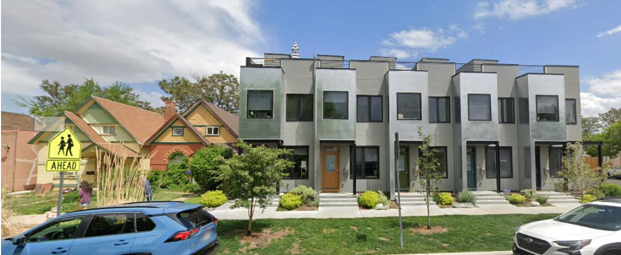
View of the properties to the east of the subject site looking east from N. Gilpin Street.
