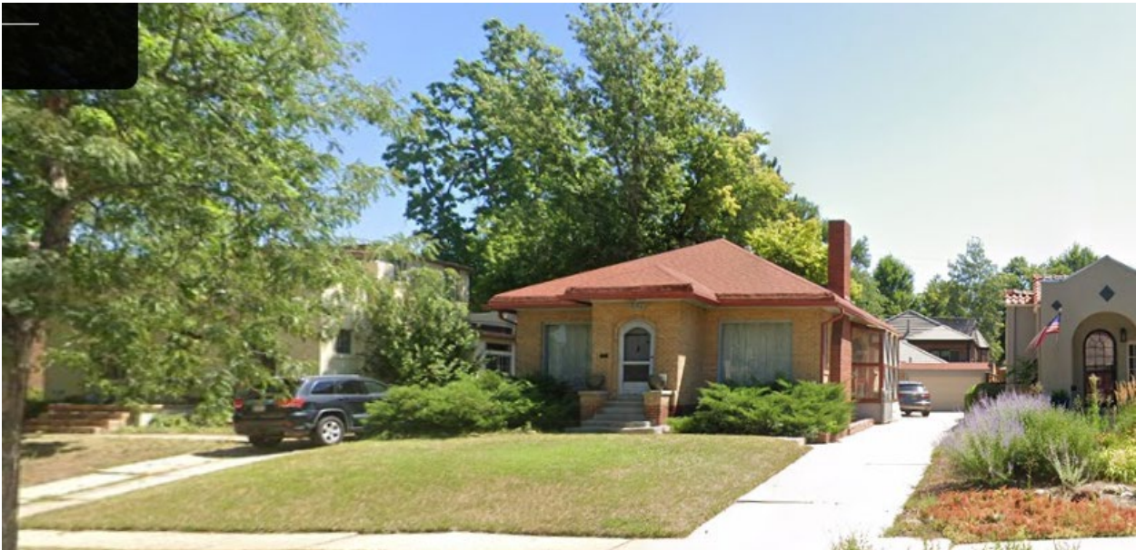
South - View of properties to the south, looking east.
