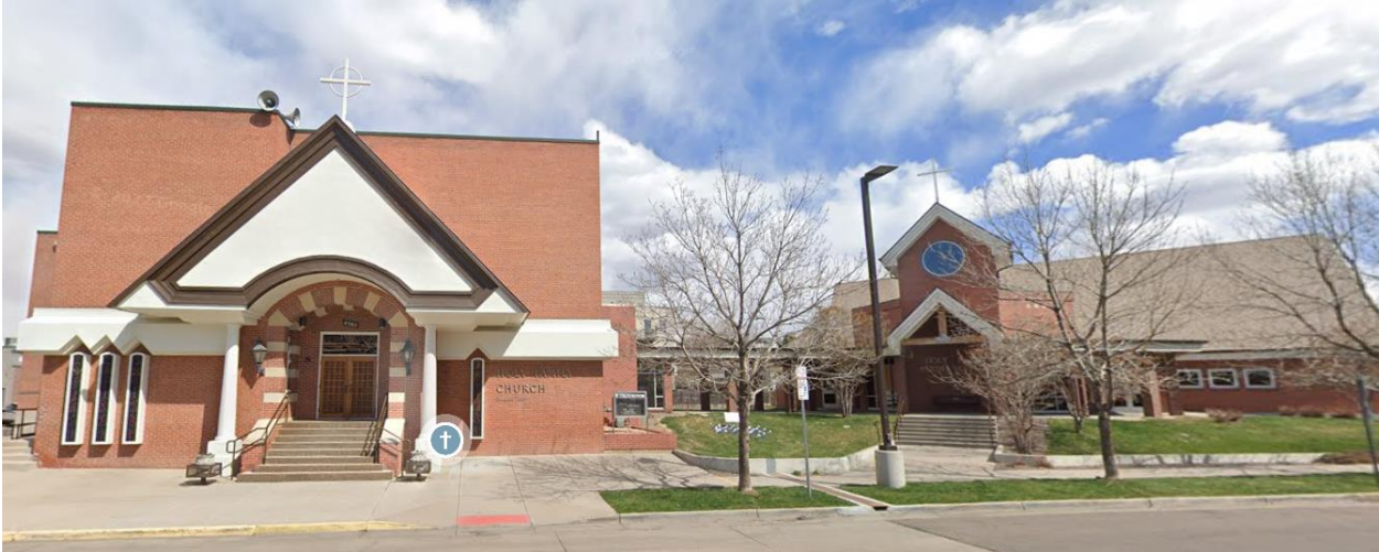
View of Holy Family Church, looking east from Utica Street.
