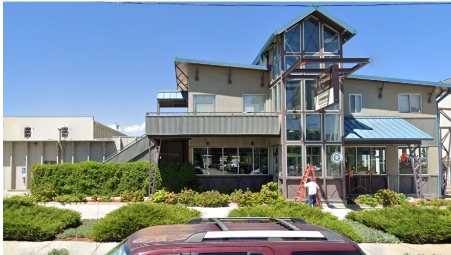
Subject site, facing west from Delgany Street
