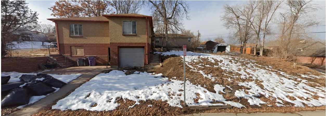
View looking west on S. Navajo Street, just north of W. Exposition Avenue – within proposed E-SU-B1 area
