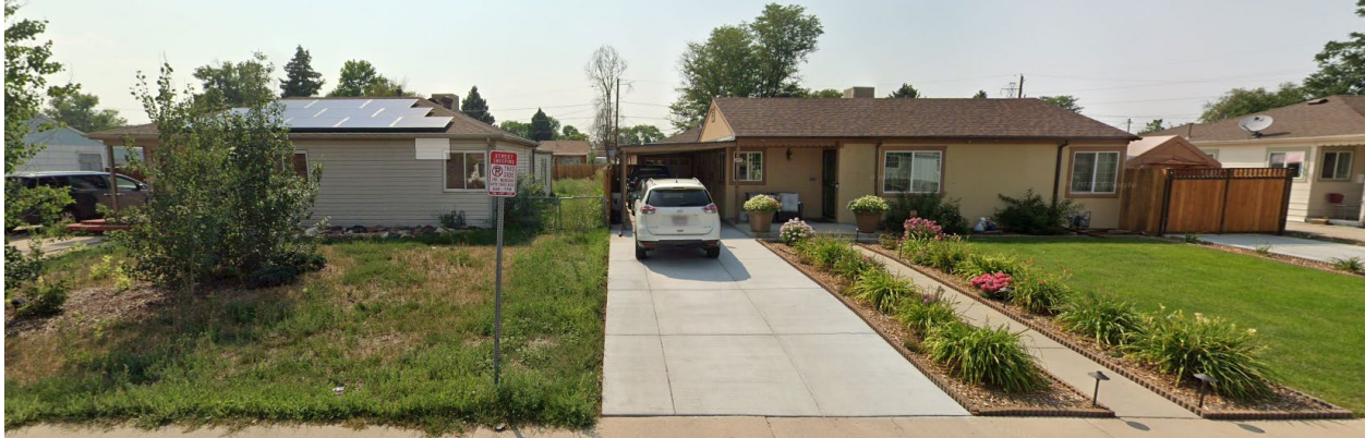
View looking west on S. Canosa Court, between W. Tennessee Avenue and W. Mississippi Ave – within proposed E-SU-D1 area
