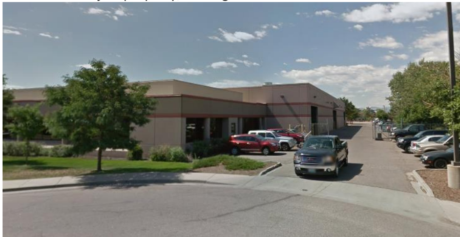
View looking southwest from 31 st Street
