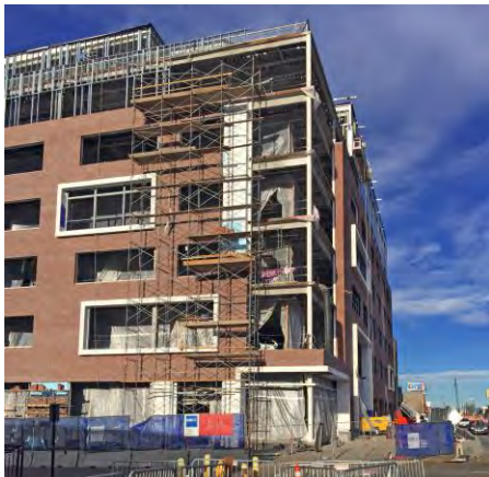
The multi-story commercial Catalyst development is under construction at 35 th and Brighton Blvd. This area would be included within both the DO-7 and IO-1 overlay districts.
