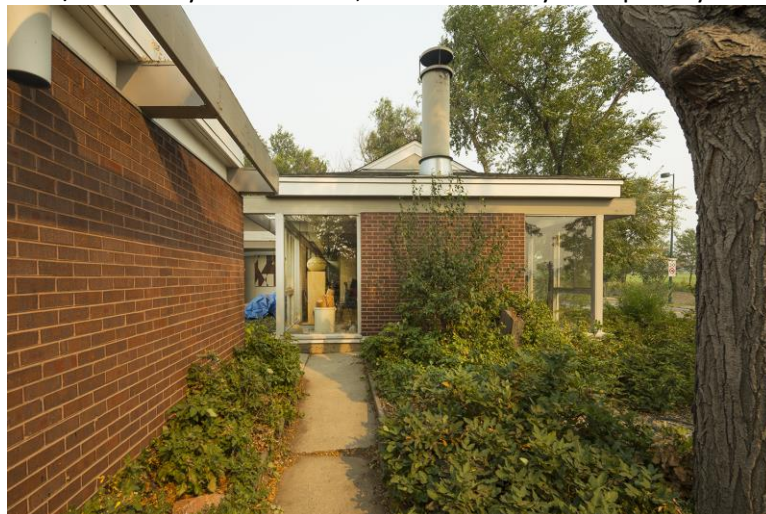
Figure 6) View of the southern wing's western end. Garage wall on the left portion of the image. Image by Paul Brokering, 2018.
