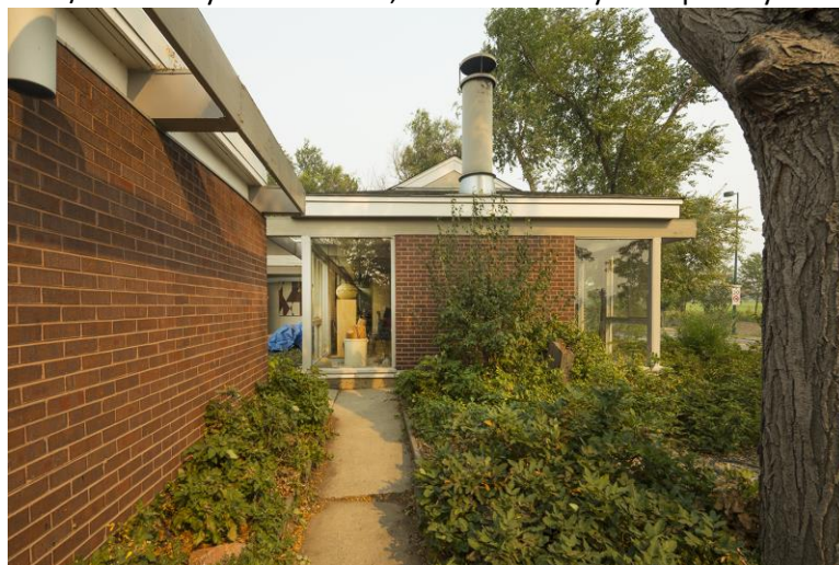
Figure 6) View of the southern wing's western end. Garage wall on the left portion of the image. Image by Paul Brokering, 2018.
