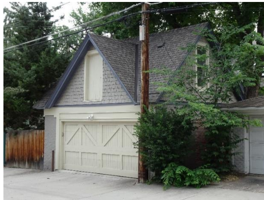
Below: Current photo of carriage house
