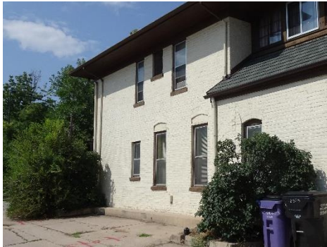
2021 photo showing partially infilled narrow and tall Italianate windows on east side of house.
