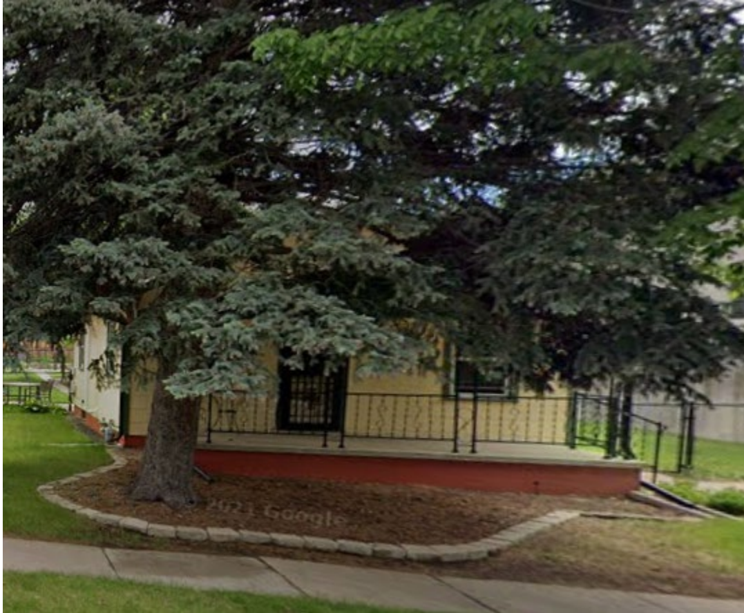
View of subject property looking east.
