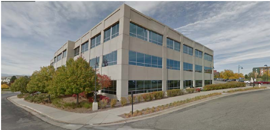
3-story office structure located directly west of the site.
