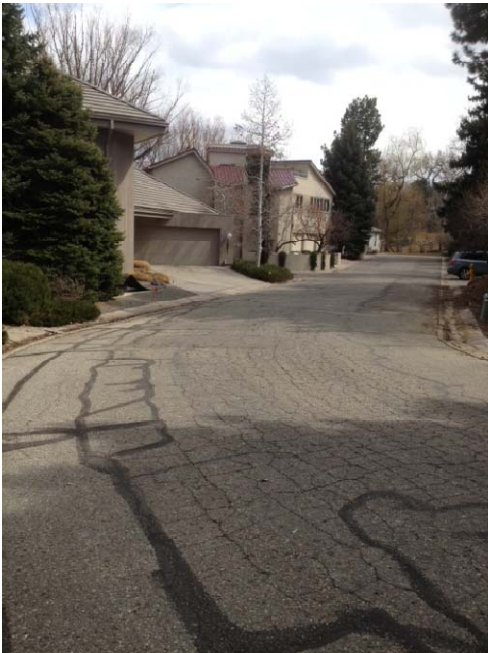
Cedar Terrace driveway and view toward east
