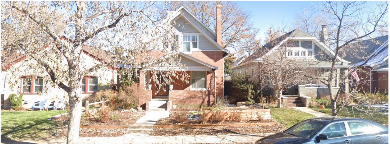
West - View of the properties to the west (across the alley).
