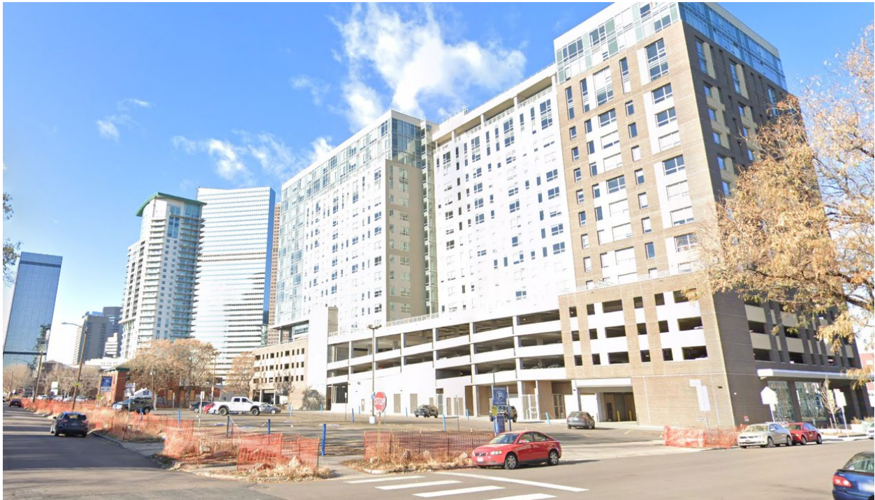
Site: Looking southwest from Glenarm Place.
