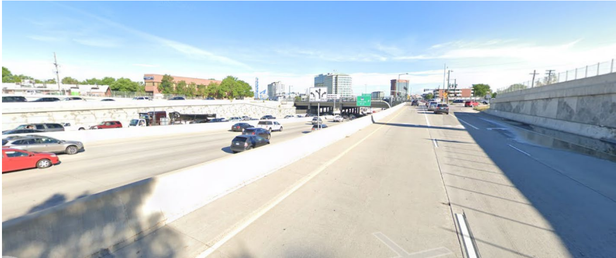
West - Looking north from Interstate 25 off-ramp to E. Evans Avenue
