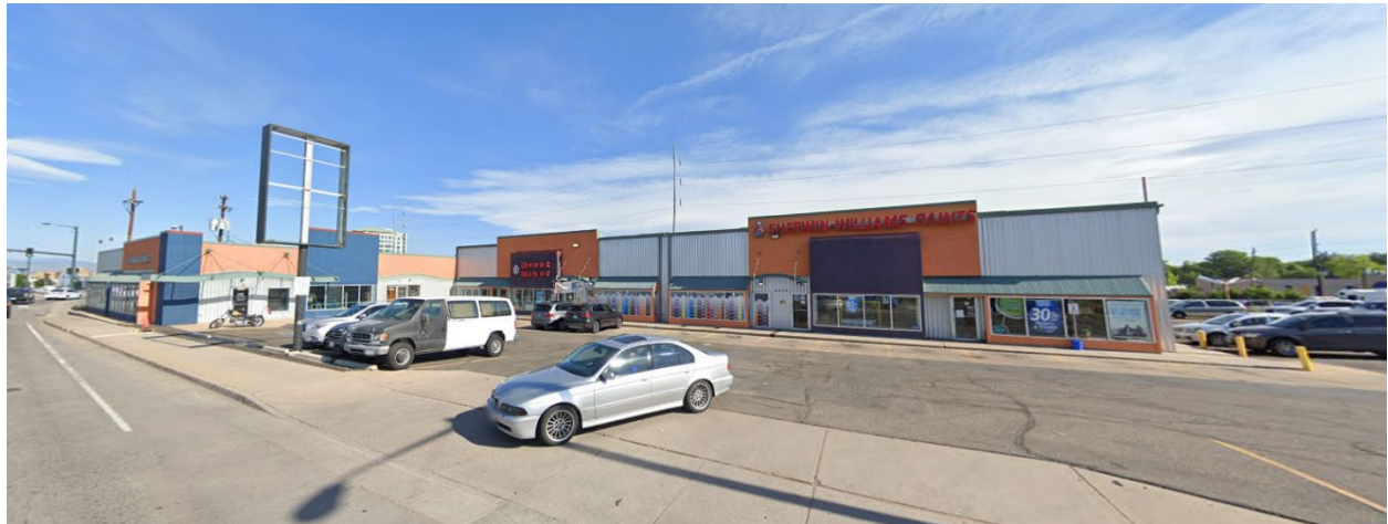
North - Looking northwest from E. Evans Avenue
