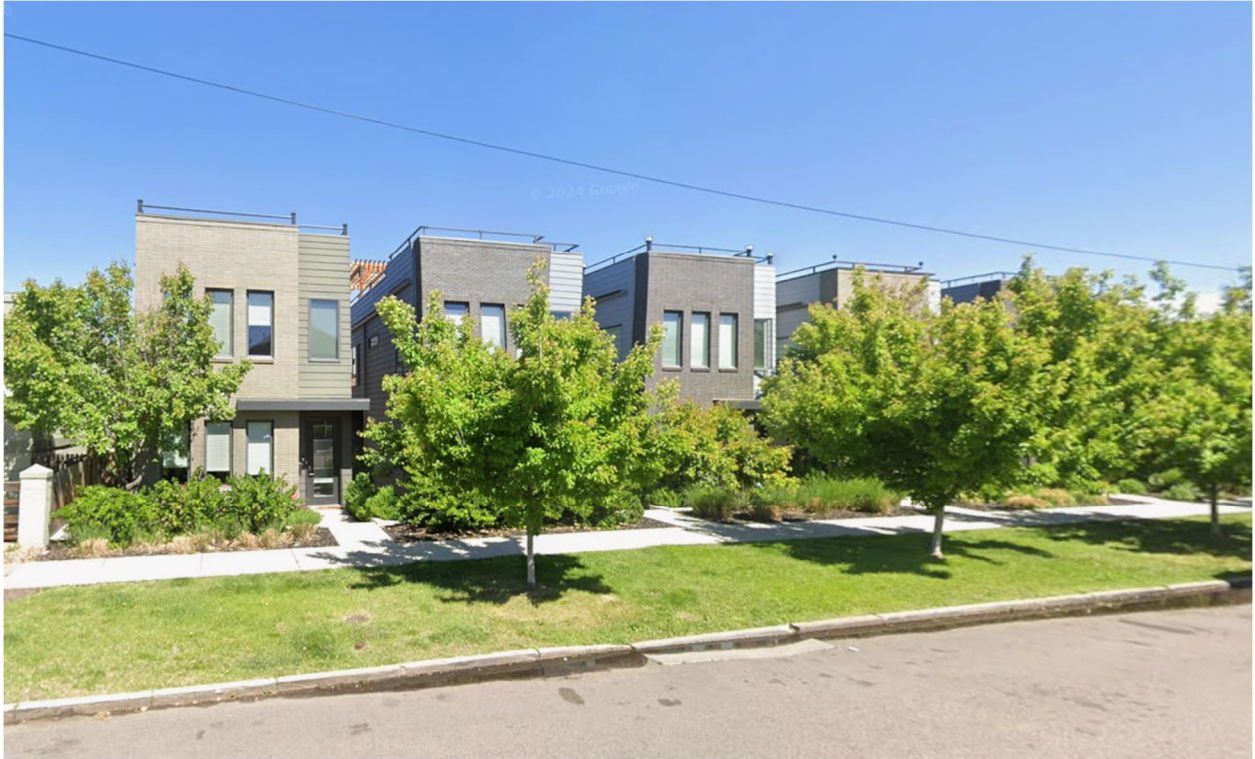
Southeast – View of the buildings to the southeast, across the alley from the subject property, looking northwest.
