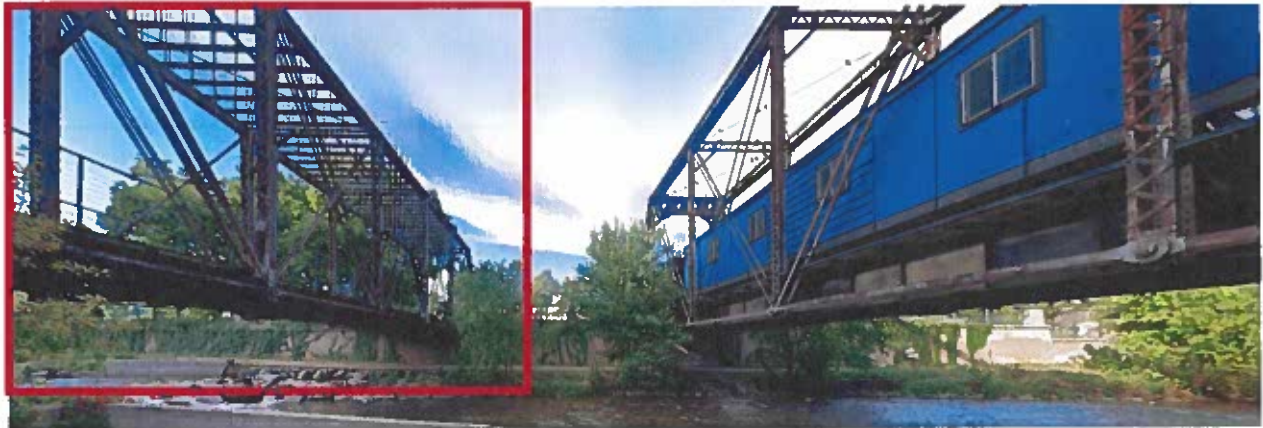
Figure 1. Bridges at the intersection of Delgany Street over the Cherry Creek.
