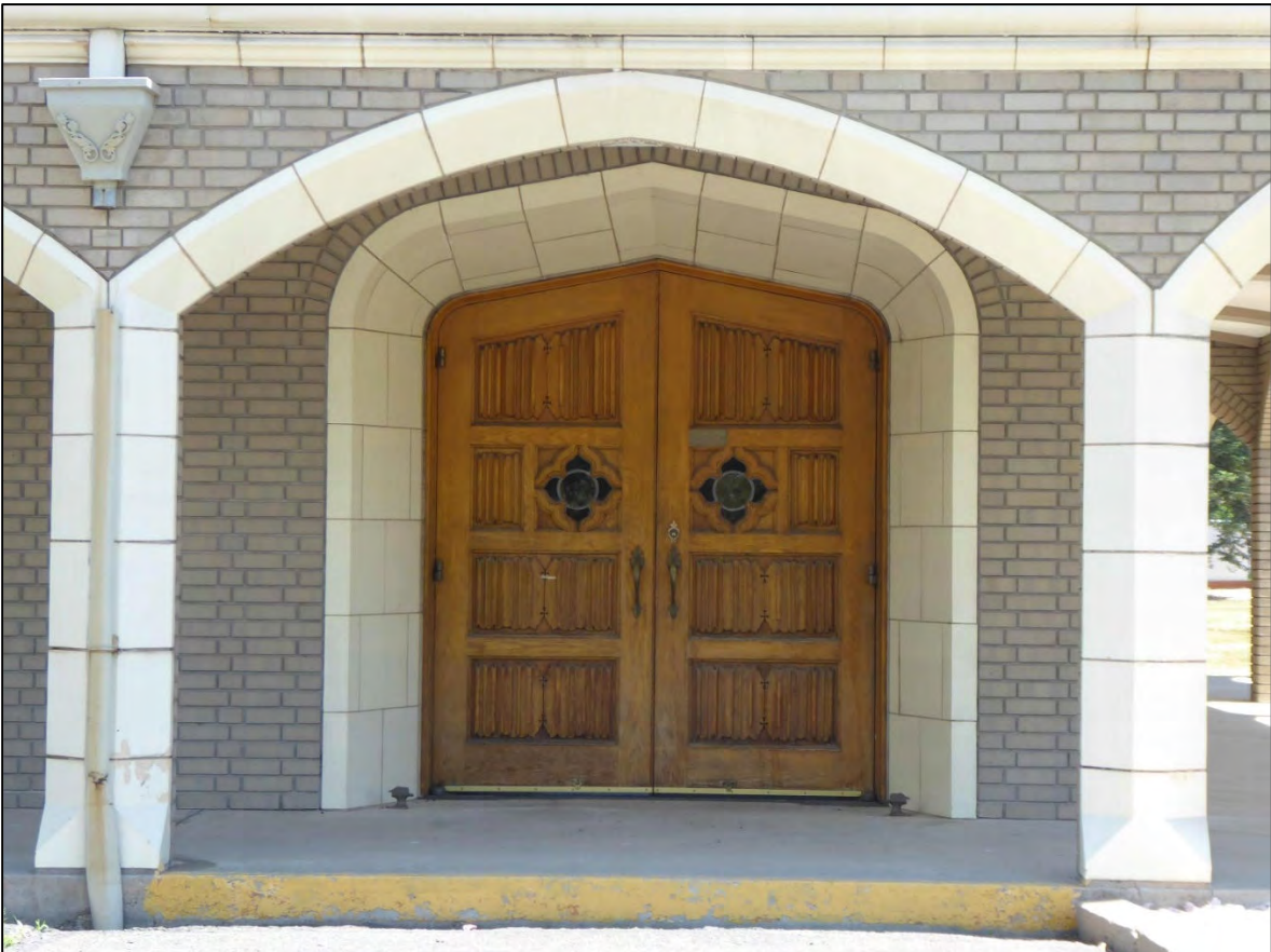
4. West double doors (hand-carved oak) and porch arcade. View east, July 2019.
