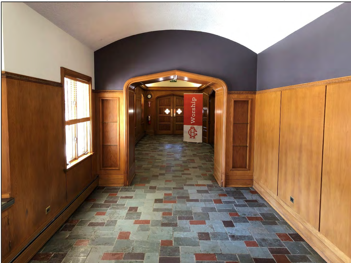
10. View down front hall toward the chapel. Note Vermont slate floor. View west, March 2020.
