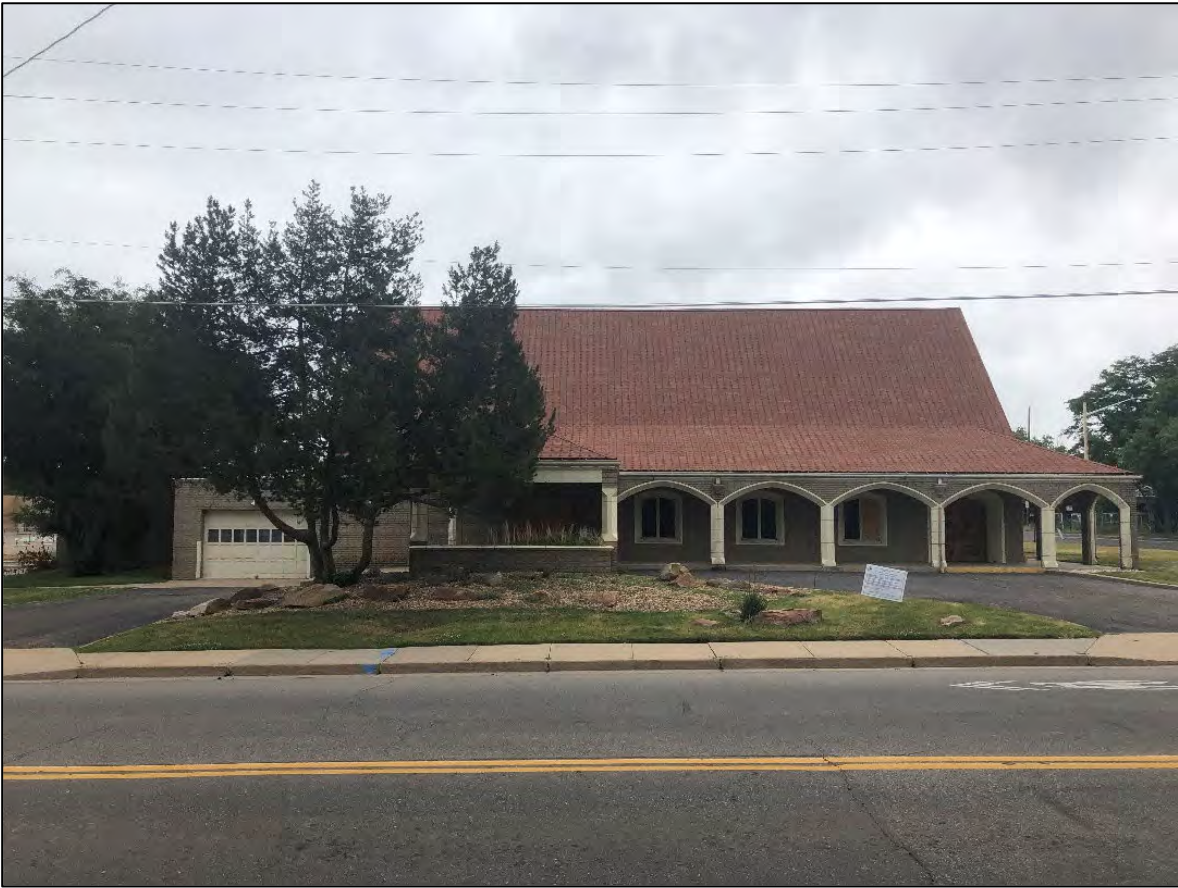
11. West wall. View east, June 2019.
