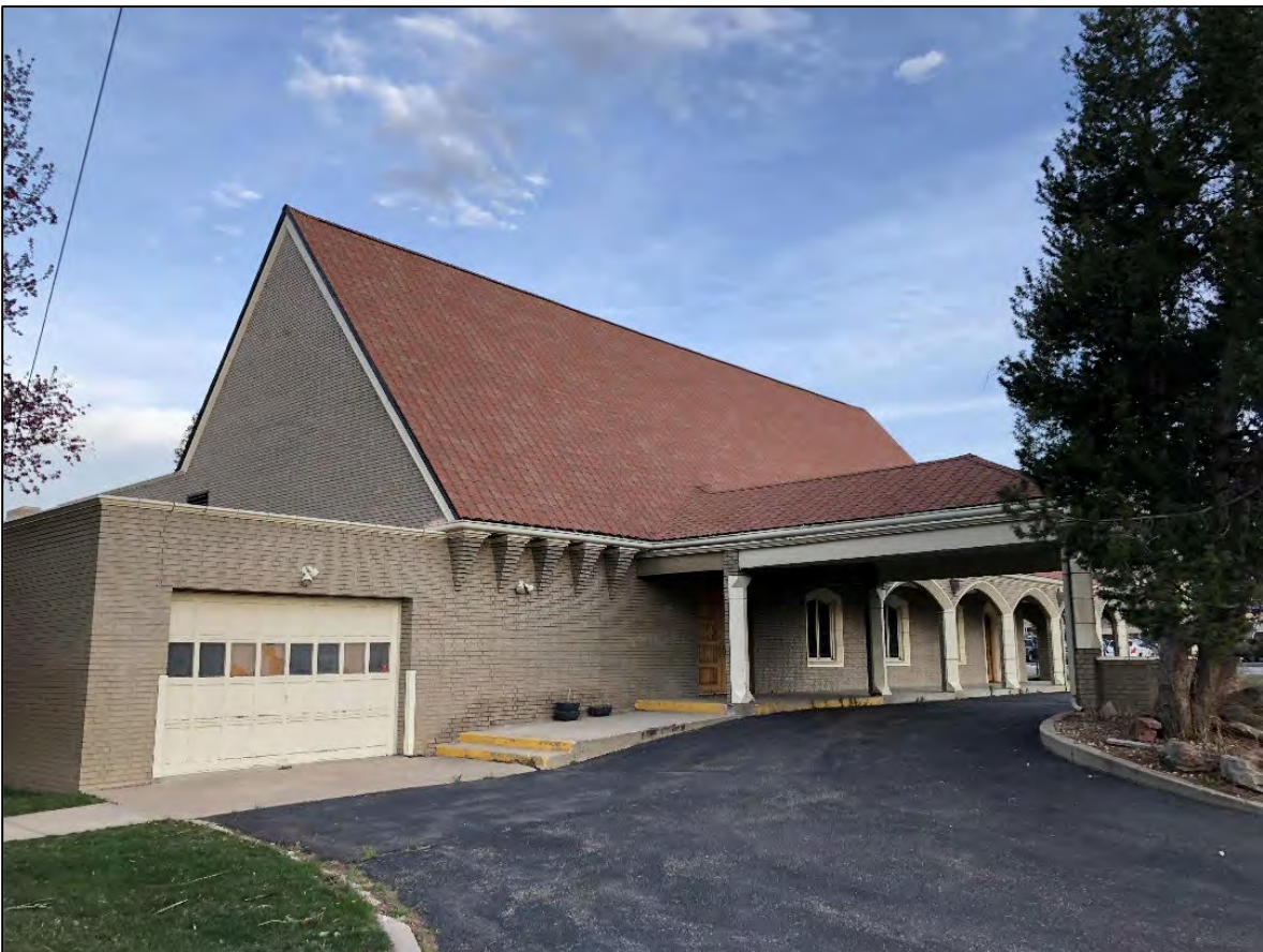
12. West wall. View southeast, April 2018.
