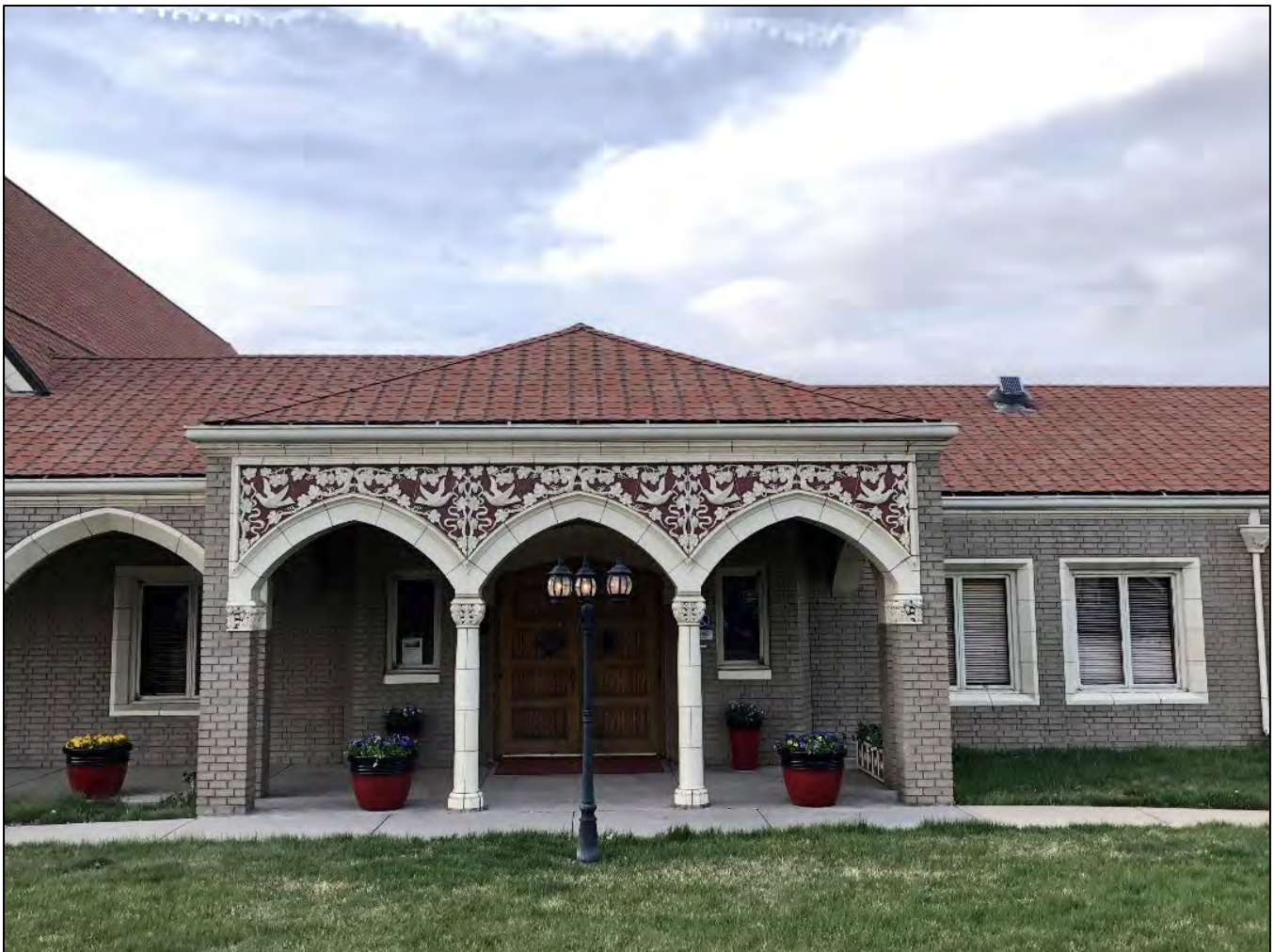
2. Front portico. View north, April 2018.
