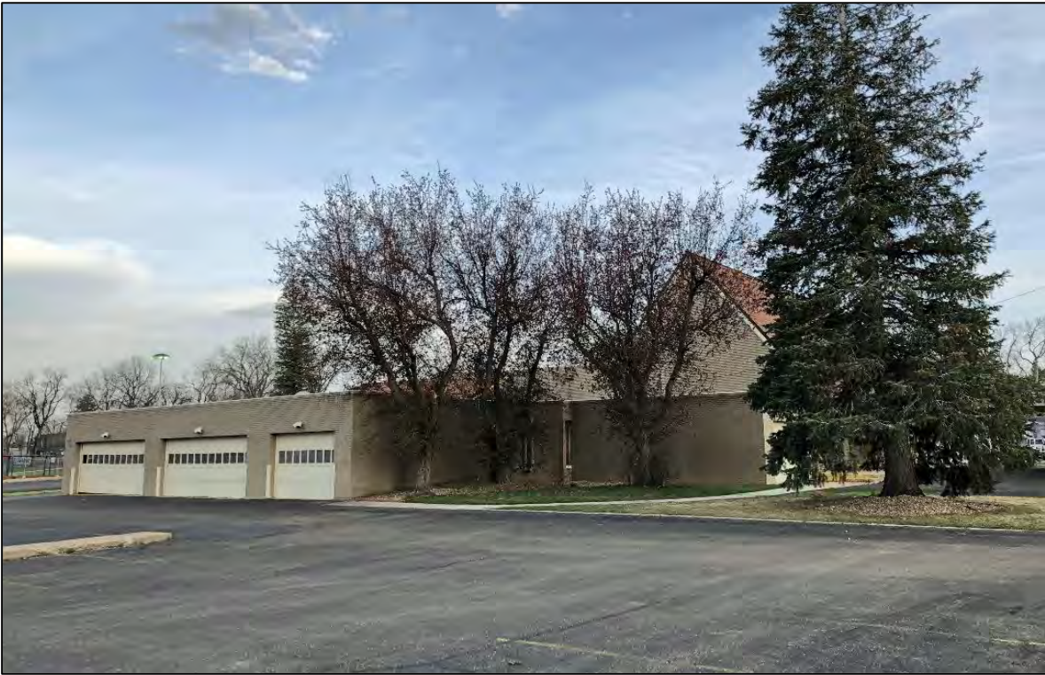
13. West end of rear. View southeast, April 2018.
