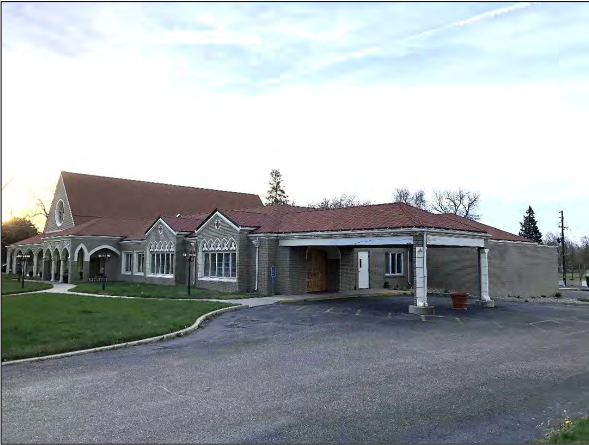
15. Three-quarter view of the front and east walls. View northwest, April 2018
