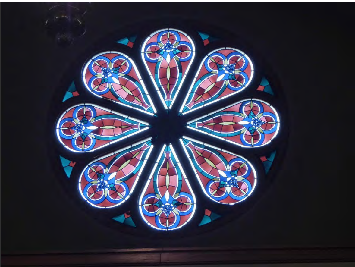
8. Rose window in south gable face of chapel. View south, May 2019.
