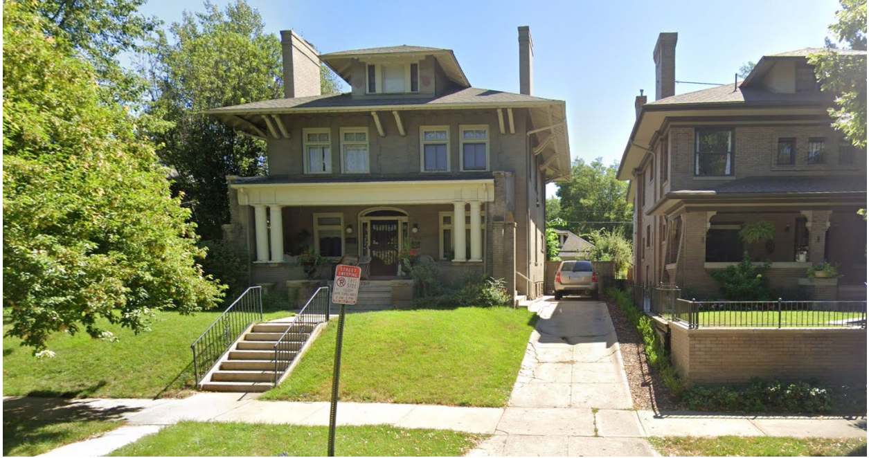
View of the property to the west, looking east.
