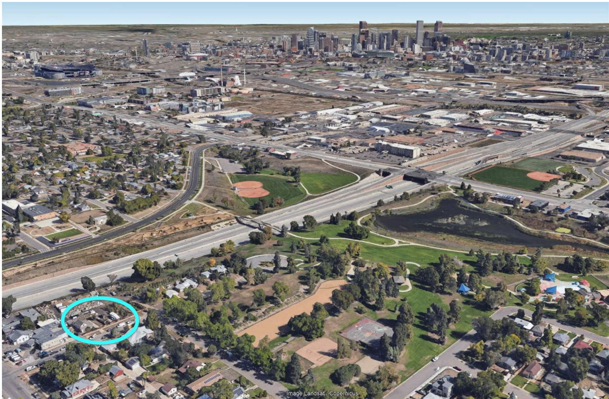
AERIAL LOOKING NORTH EAST FROM SITE- SITE CIRCLED IN CYAN
