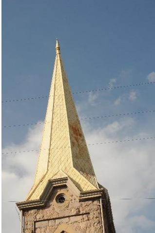
Bell tower steeple, southeast corner. Photo by Shannon Stage
