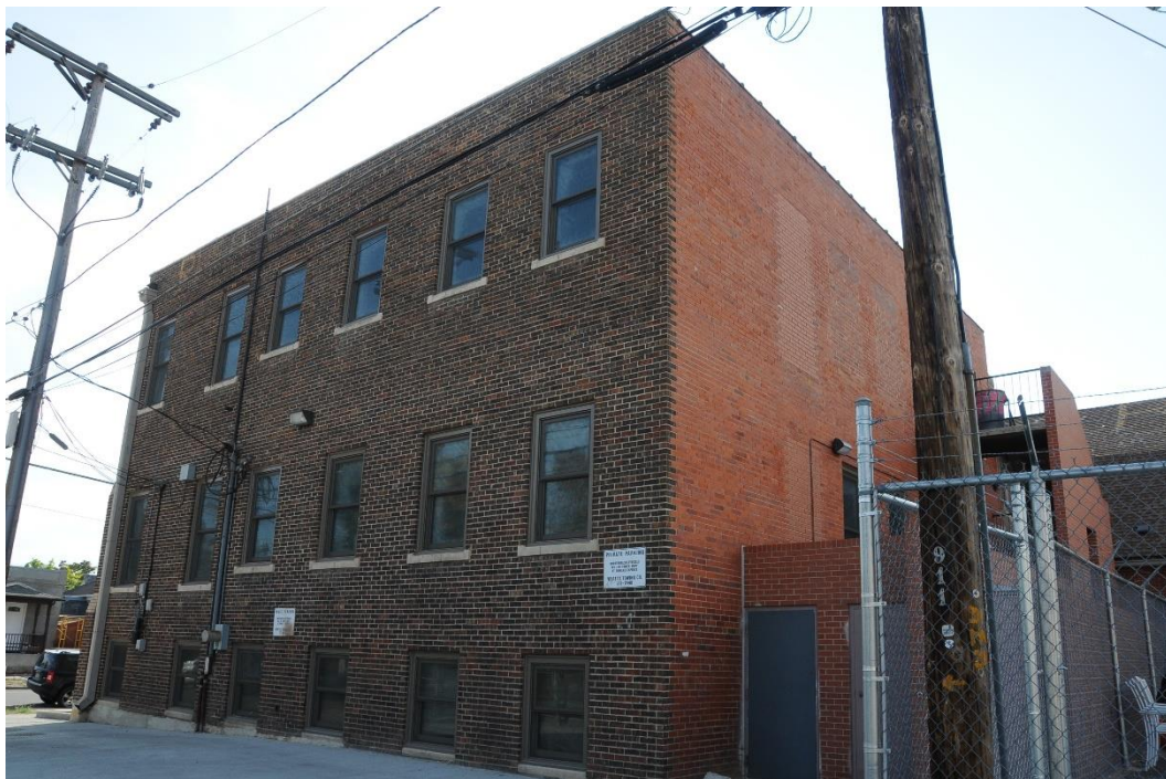
East façade of Smith's Chapel, 1923 addition. Photo by Shannon Schaefer Stage, Oct. 2020
