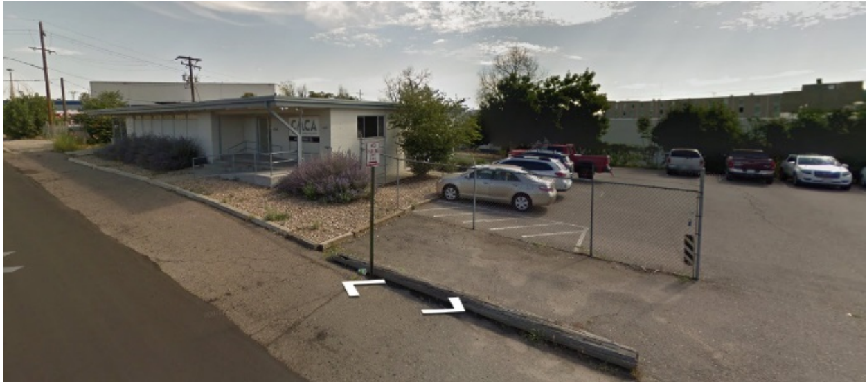
Subject Site, looking northeast
