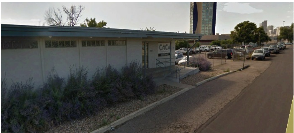
Subject Site, looking southeast
