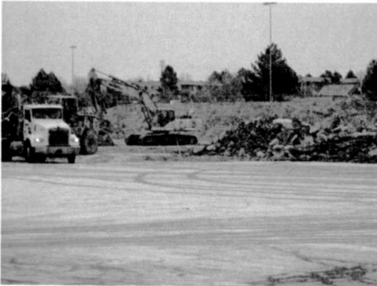
Figure 2-4: Insufficient grading or steep slopes
