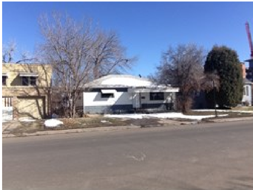
Subject Property Current Conditions: 270 South Madison Street – West View
