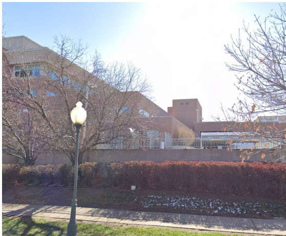
South – from E. 21 st Ave. Source: Google Maps
