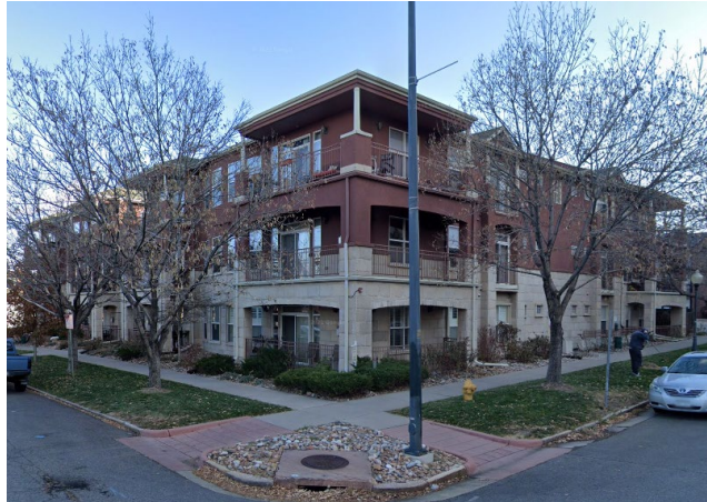
East – from E. 21 st Ave. & N. Humboldt St.
