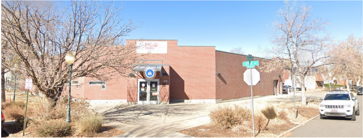
Site – from E. 21 st Ave. & N. Humboldt St.
