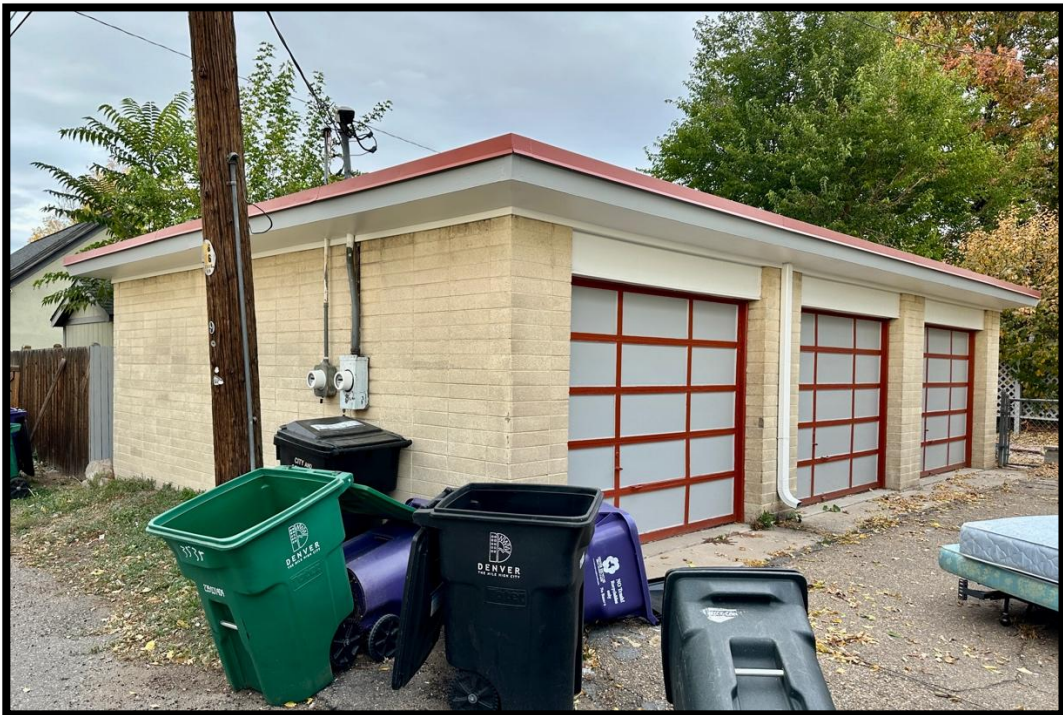
Detached Garage, View to the Northeast
