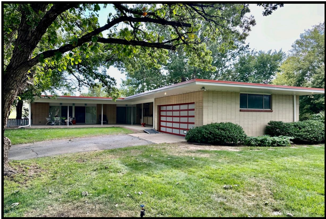
Rear of the Harris-Cousins House, View to the Southwest
