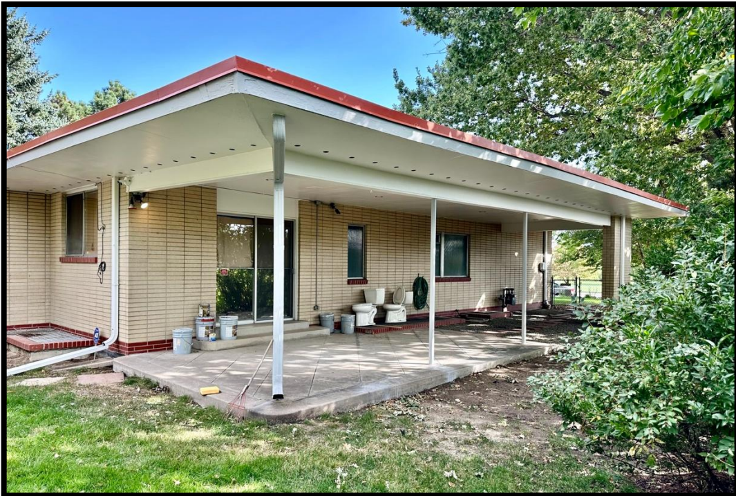
The West Porch, View to the Southeast
