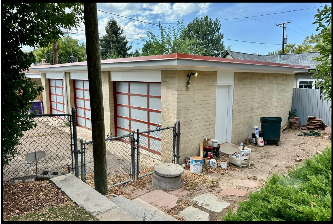
Detached Garage, View to the Northwest
