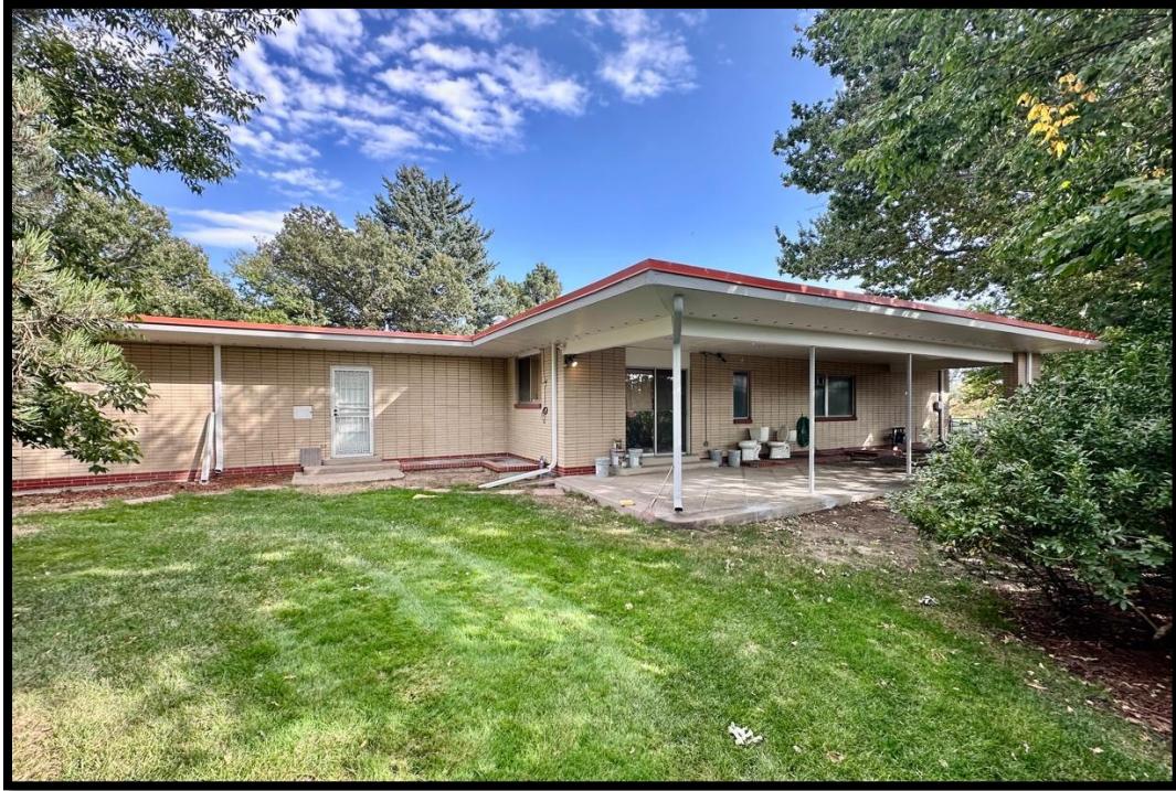
West Side of the Harris-Cousins House, View to the Southeast
