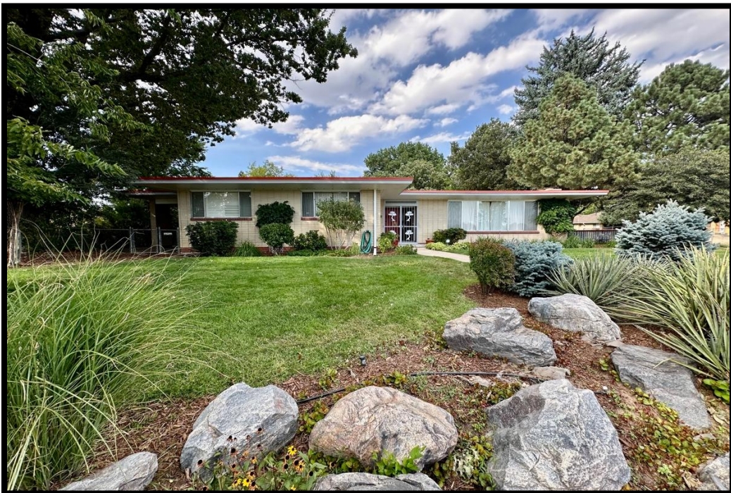
Front of the Harris-Cousins House, View to the North
