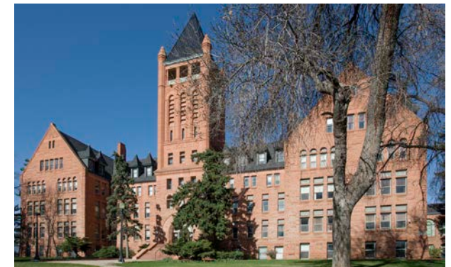
From top to bottom: Theater and Administration Building
