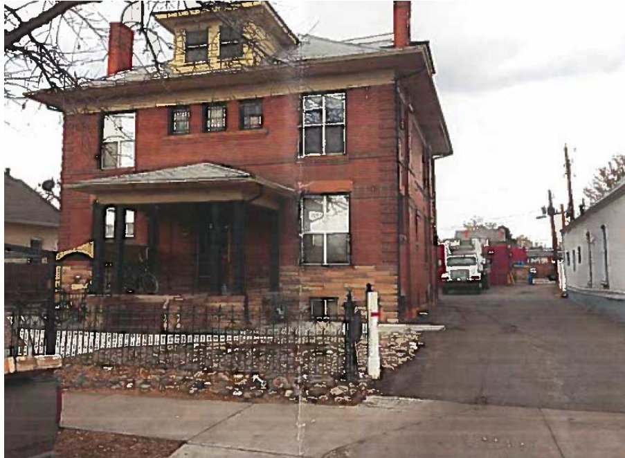
View of the Remaining Building defined in PUD-G 16 from Tejon Street looking west showing existing drive aisle on north side of subject property.
