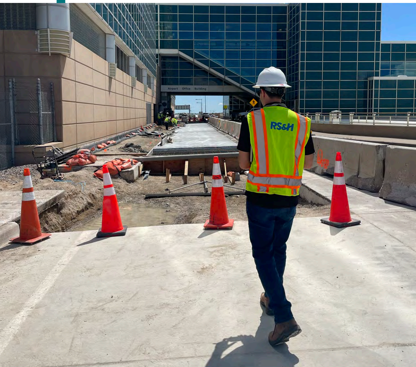
RS&H's Jorge Caraveo monitoring construction on the DEN Level 5A Roadway Rehabilitation Project.
