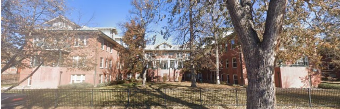
Properties to the east, as seen from W Fairview Pl
