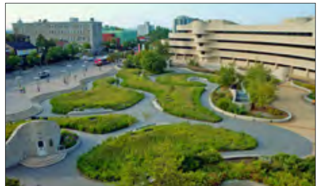
The NWCC Transit Station will have large planting areas, a dense tree canopy, and public art.
