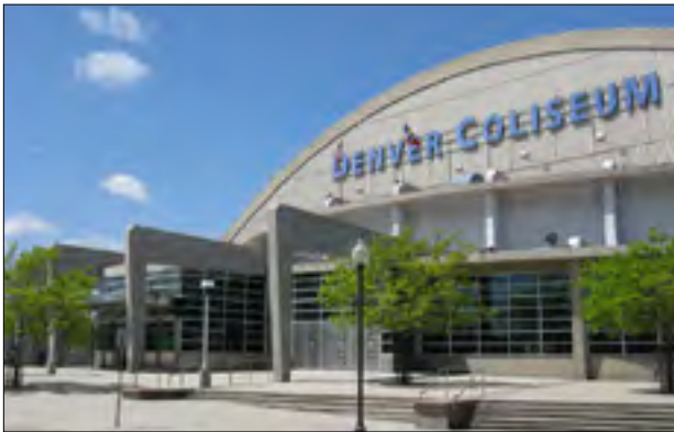
The Denver Coliseum is a potential facility for reuse to support the NWC.
