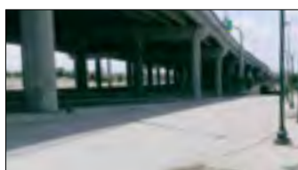
2000 Elevated I 70 and 46th Avenue reconstructed west of Brighton Blvd.
