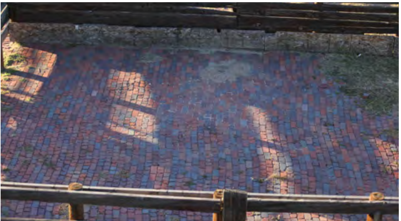
Historic brick pavers
