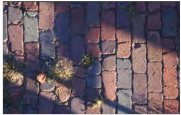
The brick pavers in the existing yards are an important historic artifact that will be reused in the new NWC.
