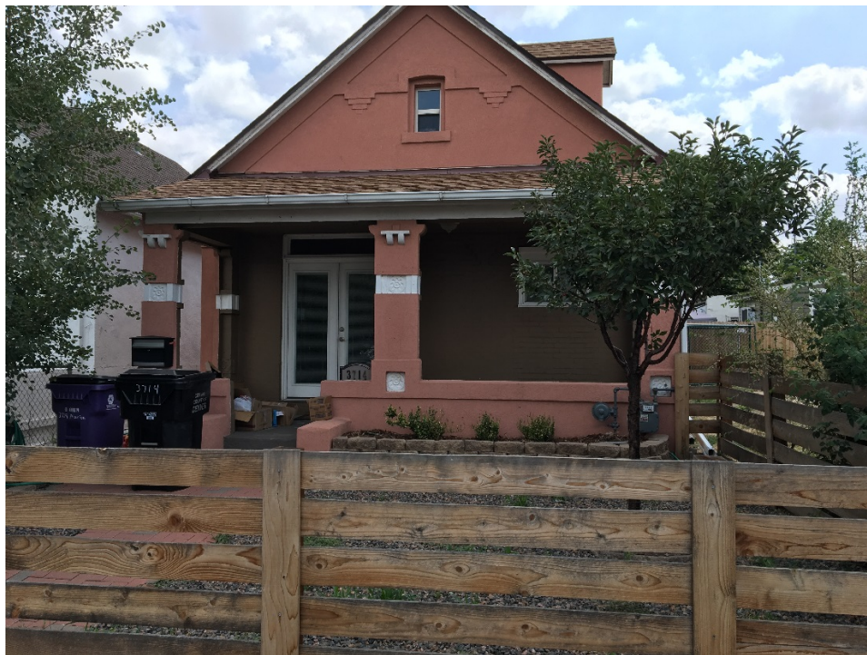
View of the single family home adjacent to and north of the subject site.
