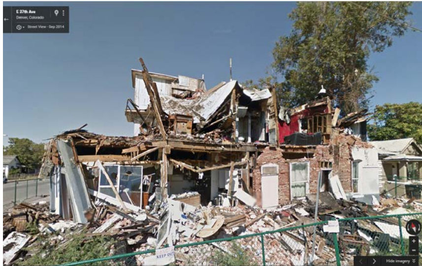
The ruins of the former structure as it appeared in August, 2014. Source: Google Street View
