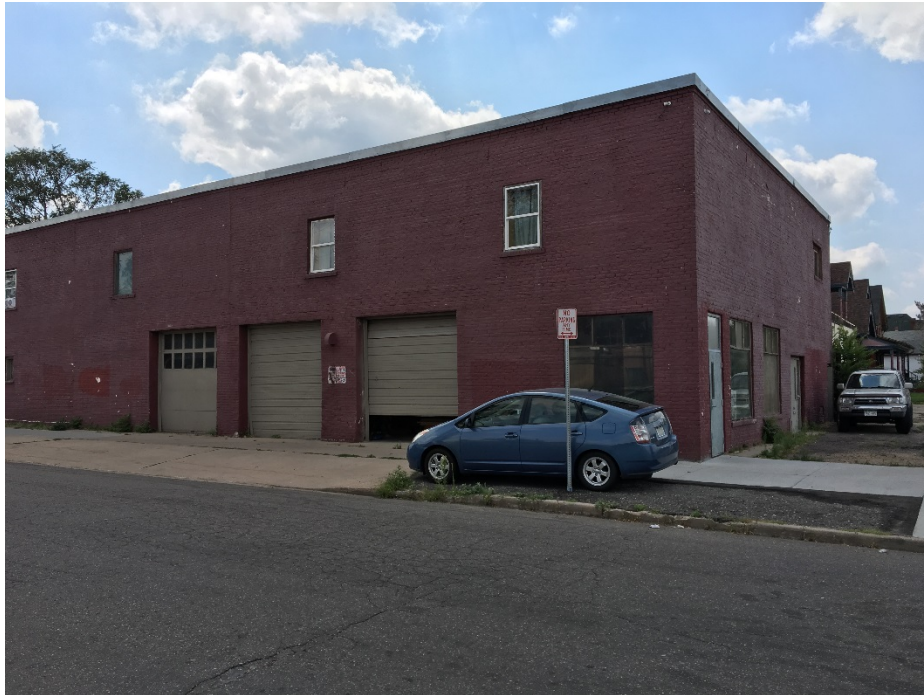
This industrial building is located south of the subject site, across 37 th Ave.
