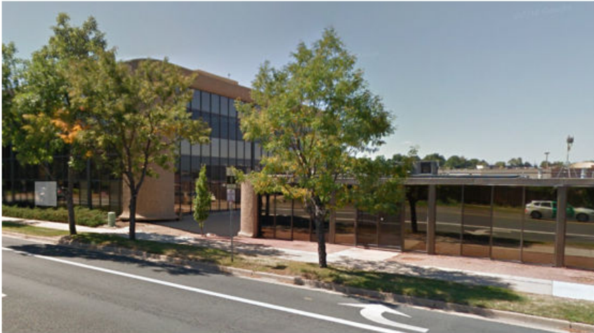
Subject Site, looking west
