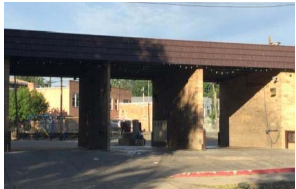
East – View from Speer Boulevard of commercial carwash facility in the foreground with the subject property (school and church) visible in the background.
