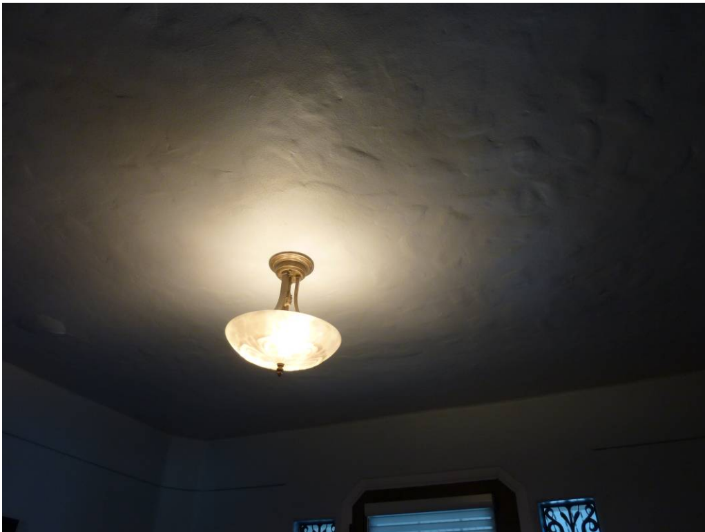
Fig 3: Textured Ceiling in Dining Room
