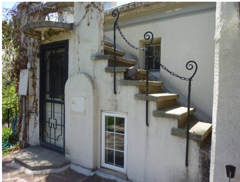
Back Staircase Detail
