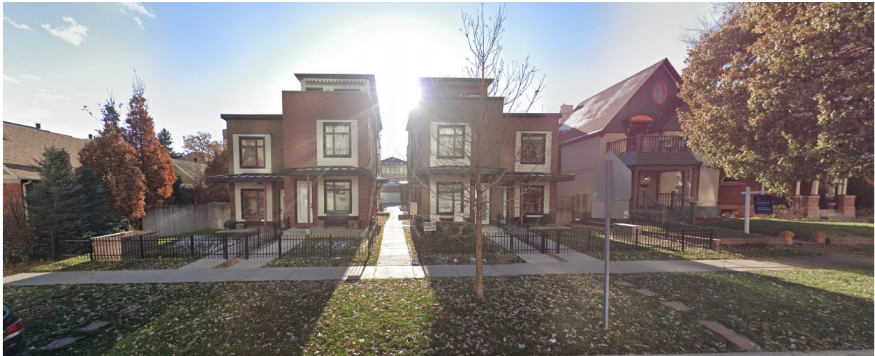
Northwest – from Glenarm Place, looking southeast.
