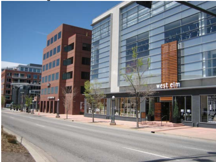
The site at 1 st Avenue
