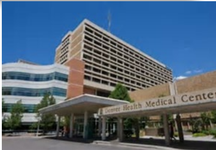
1997 Denver Health and Hospital Authority
