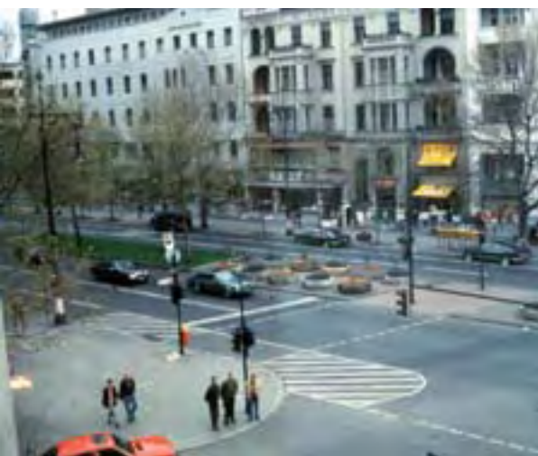
Bulb-outs, brightly-striped crosswalks and landscaping help to make this intersection in Germany more pedestrian friendly.
