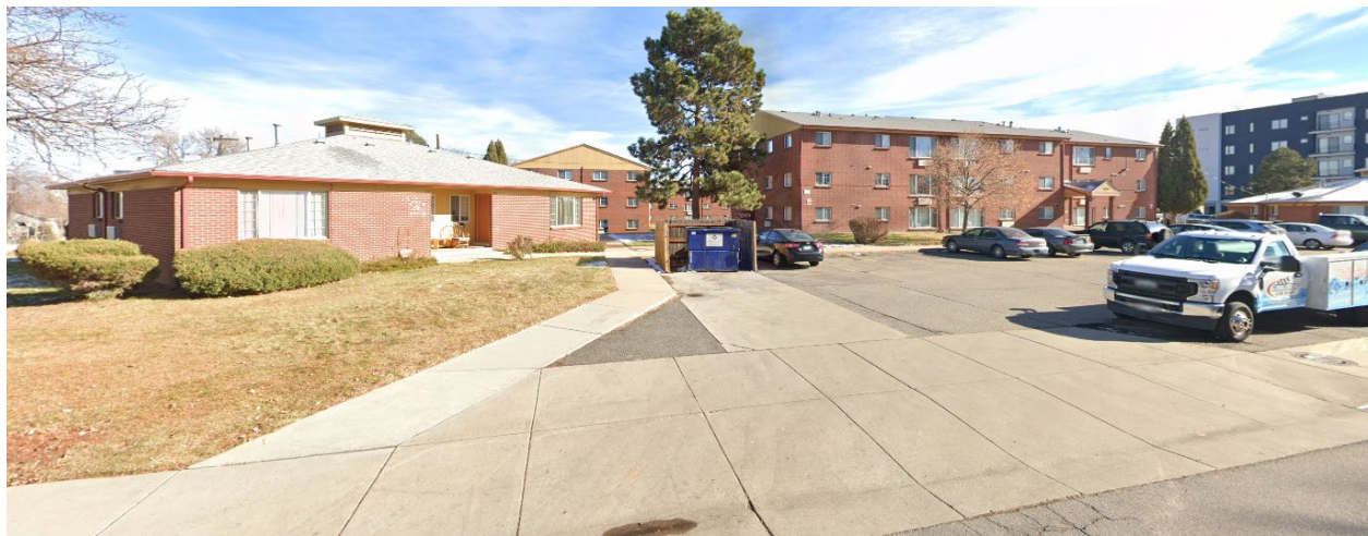
Site – The subject property from North Hooker Street, looking east (Source: Google Maps)
