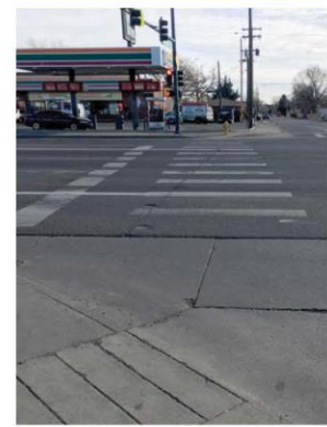
VIEW A: View looking east along Kentucky Avenue of the long pedestrian crossing distance
