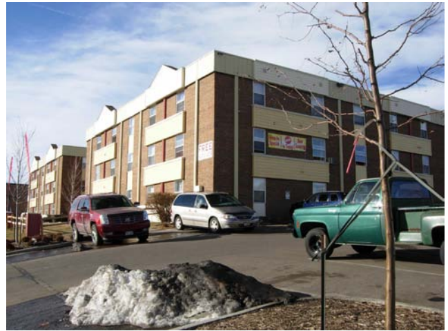
Low-rise multi-unit south of the subject property
