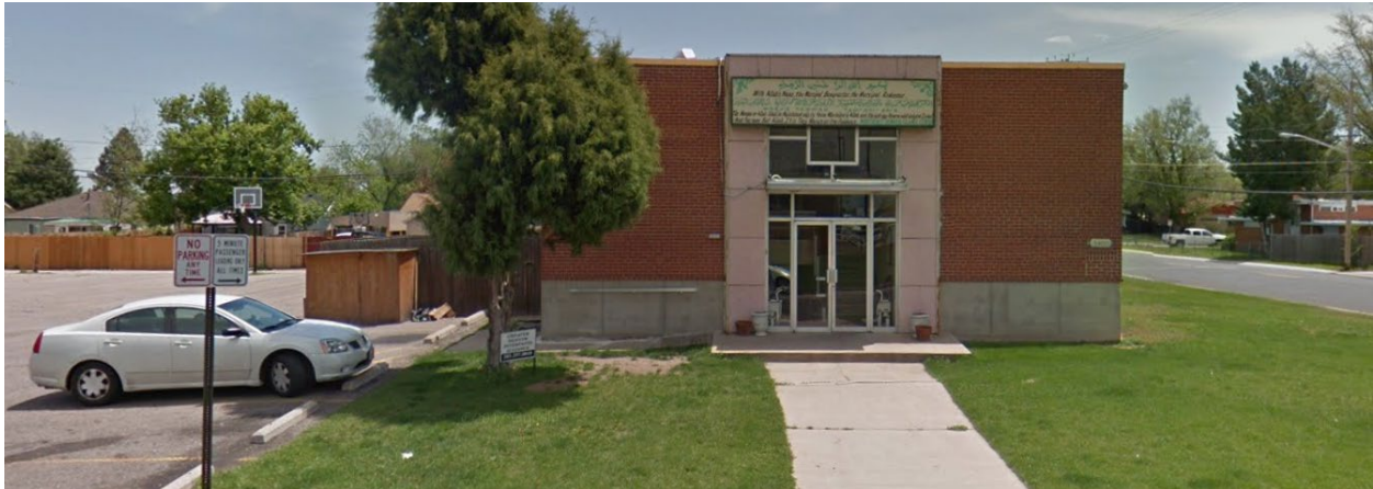
Place of Worship institutional building across Albion from subject site, looking east.
