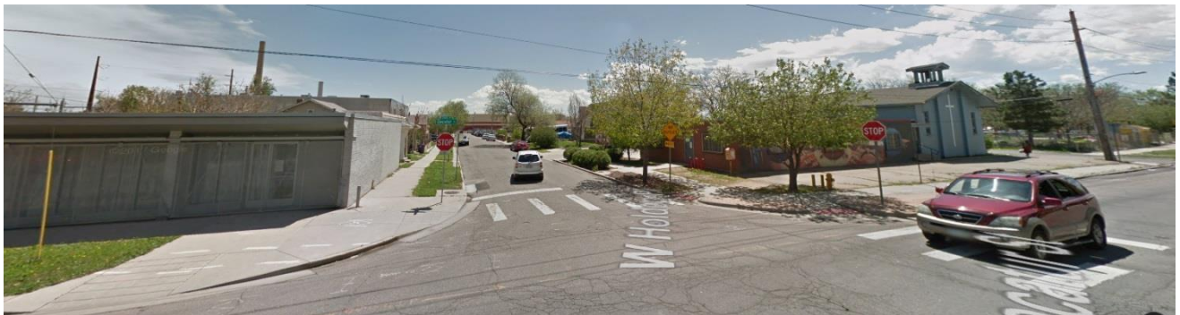
Sun Valley Youth Center, commercial kitchen and other uses east of the site, across Decatur St.
