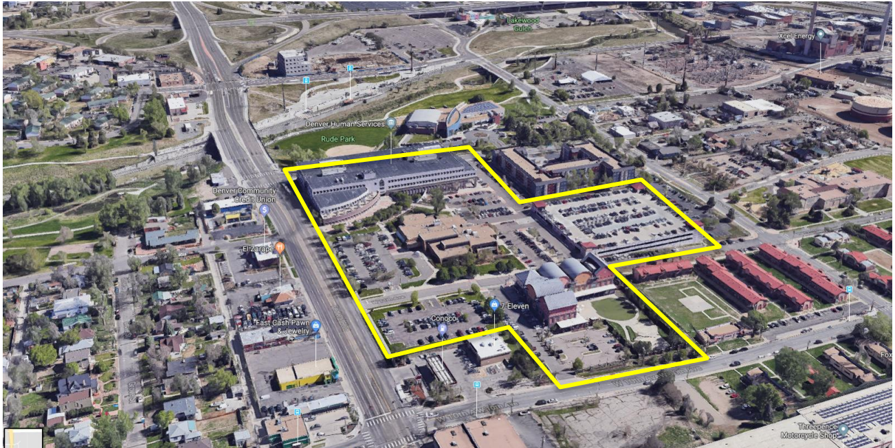
Aerial View of subject site and surrounding development, looking northeast along Federal Blvd.
